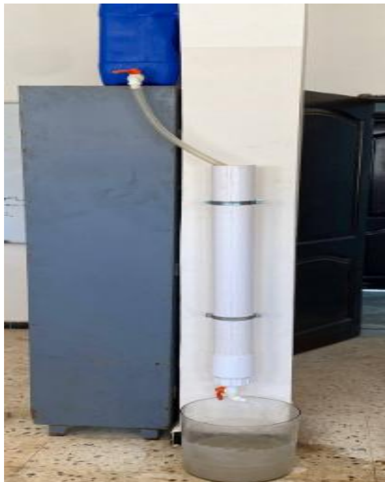
Figure 5. The Modified Sand Filter (MSF) with biomass of Sawdust (SD).
