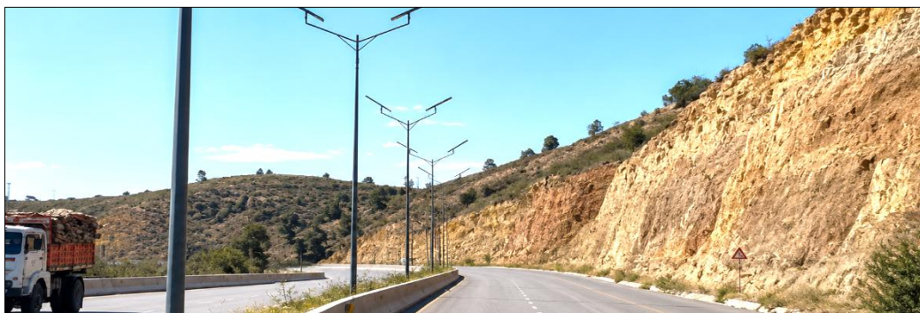
Figure 1. Cut slopes along the Al-Naqaza mountain road, Al-Khums.
